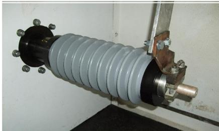
The project involved the renewal of 21 new VMAG 25 high voltage circuit breakers (HVCB's), associated busbar supports, bus section through wall bushing and voltage transformers within each busbar chamber. The interface between the existing Alstom Micom Protection relays and VMAG 25 CB was modified and re-commissioned to ensure compatibility and correct tripping functionality.
